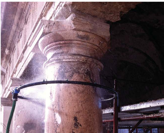
foto work in progress
