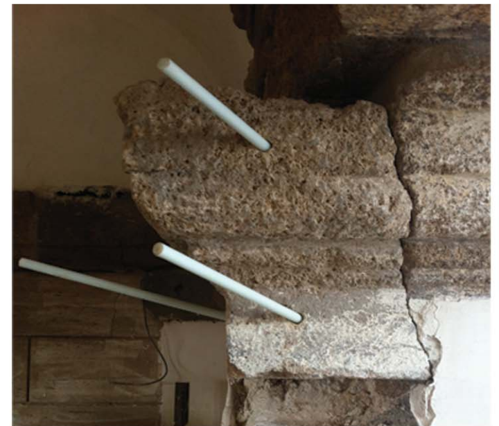
foto work in progress
